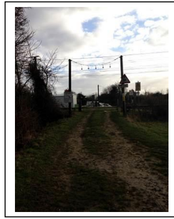
Down side crossing approach
